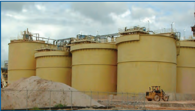
200 HP mixers operating on 59' CIL tanks.
