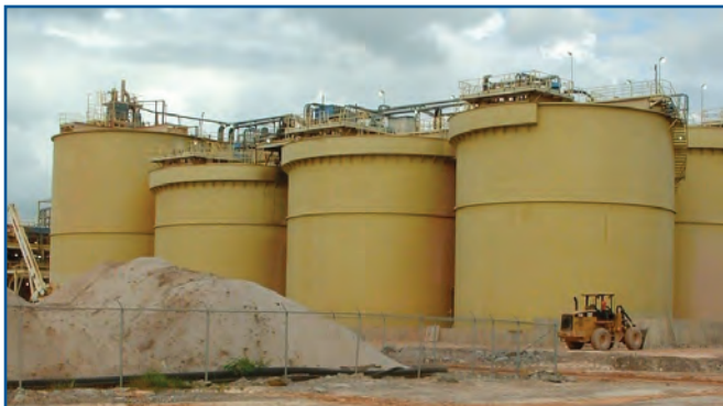
200 HP mixers operating on 59' CIL tanks.
